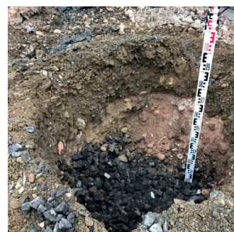
Figure 20: Left: concept drawing of the insulating bore pile wall – horizontal section [10]; Right: mock-up of bore pile filled with foam glass gravel
