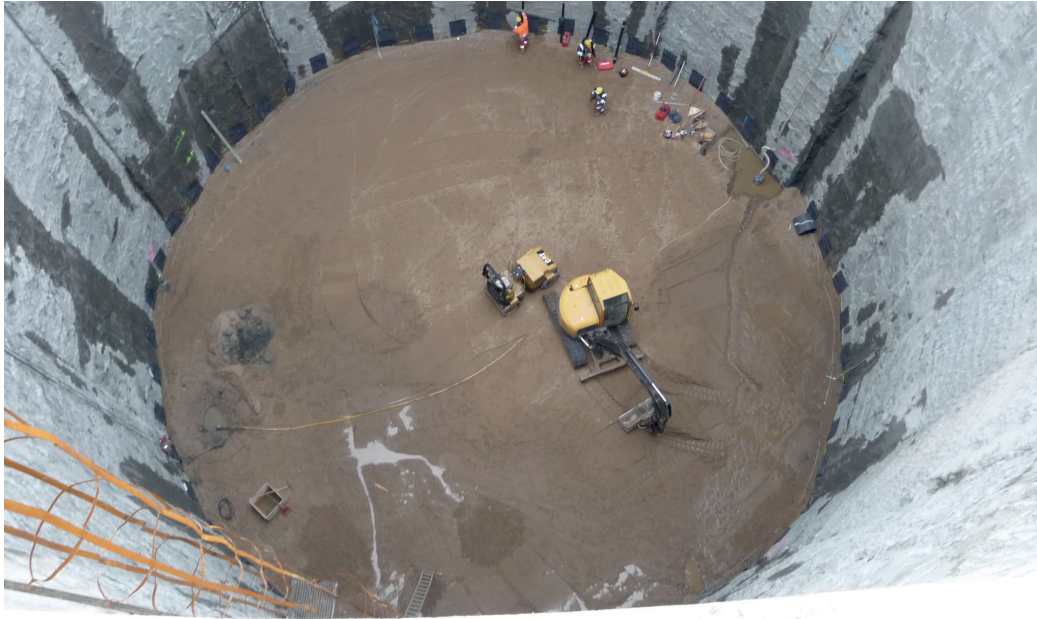
Figure 8: Finished elliptical diaphragm wall shaft - top view [©PORR]
