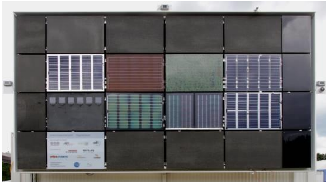
Figure 4: SFL BIPV test facade
