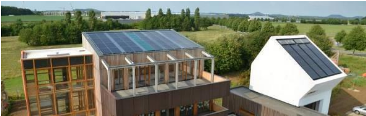
Figure 14: District of tomorrow BIPV test facility
