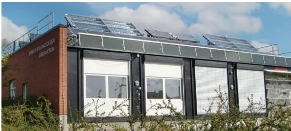
Figure 18: Lund University outdoor BIPV test facility
