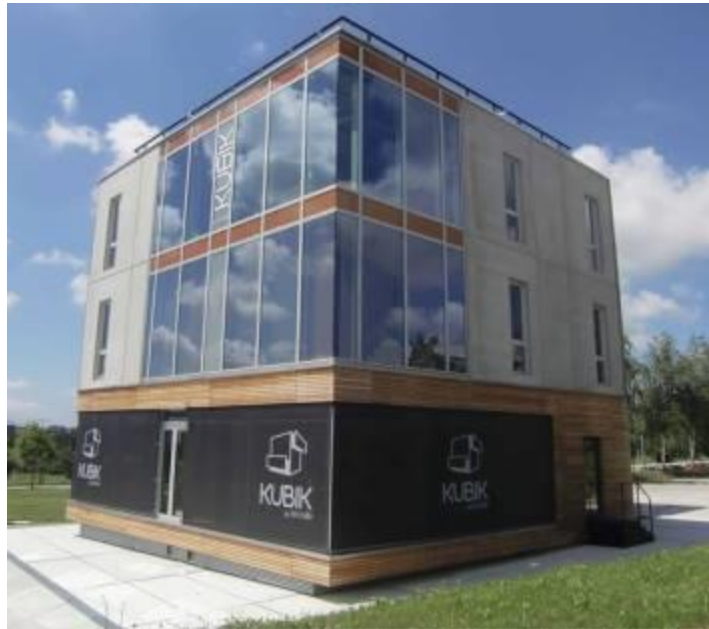
Figure 16: Tecnalia KUBIK BIPV outdoor test facility
