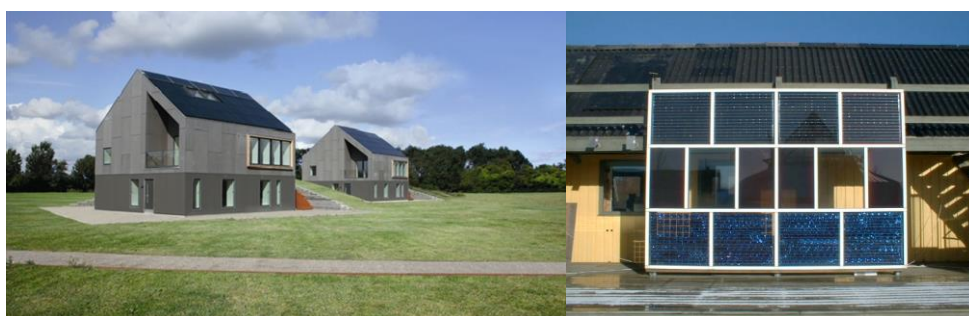
Figure 20: DTI BIPV Test facilities
