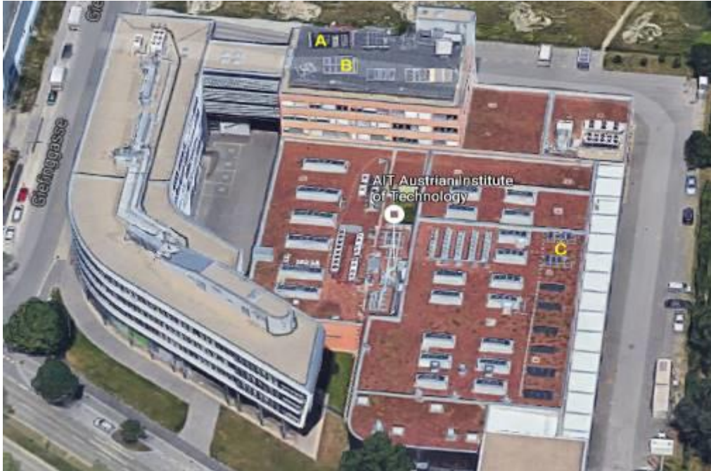
Figure 2: AIT TechBase roof outdoor test stands
