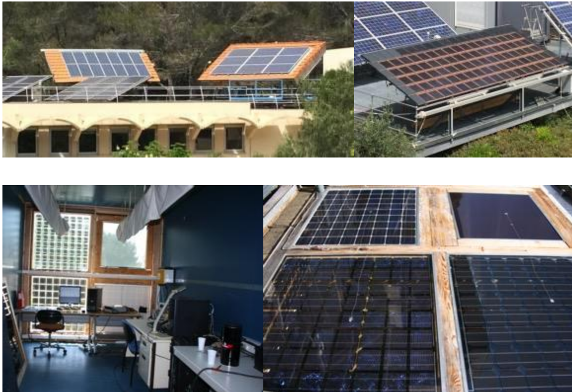
Figure 8: CSTB Test facility
