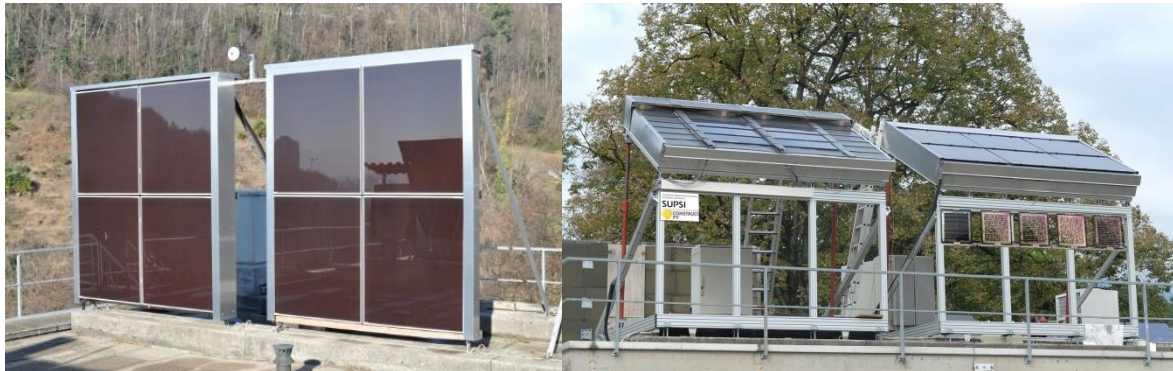
Figure 19: SUPSI BIPV Test facilities
