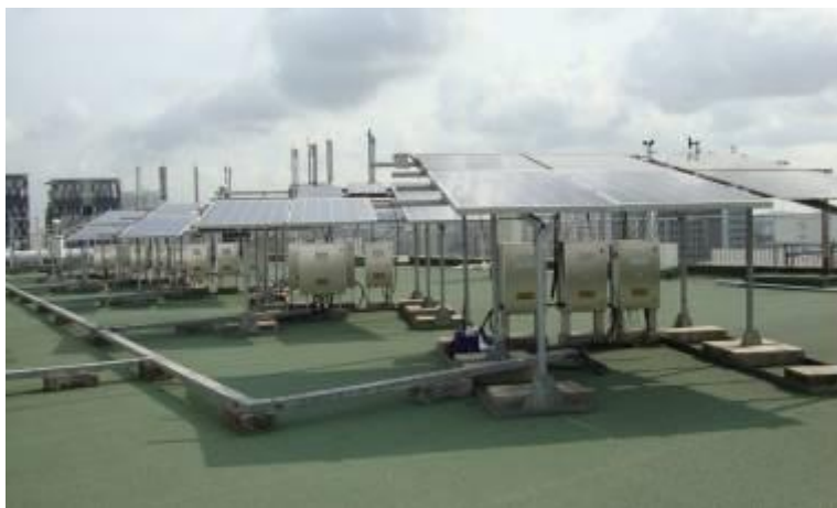
Figure 11: SERIS outdoor test facility
